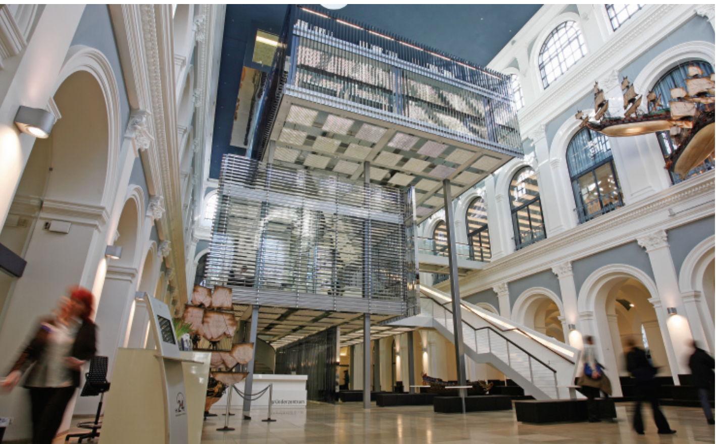
The 15,000-square-foot, five-story steel and glass structure was constructed elsewhere, broken down and then reconstructed on-site. Stairs and a footbridge connect the new structure to the original building.
